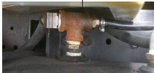
Fuel Lines From Tank
